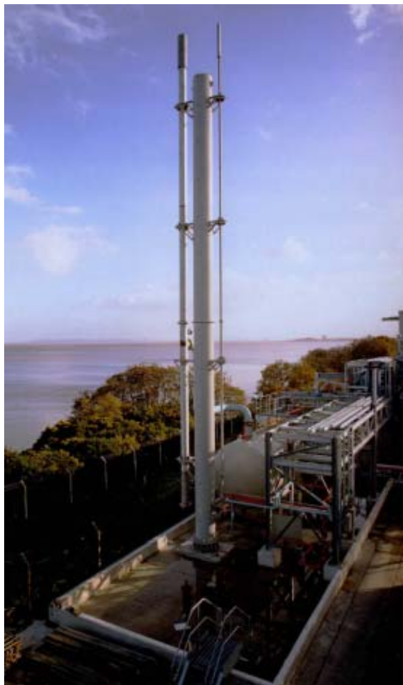
Figure 4 Quench tank site and installation.
