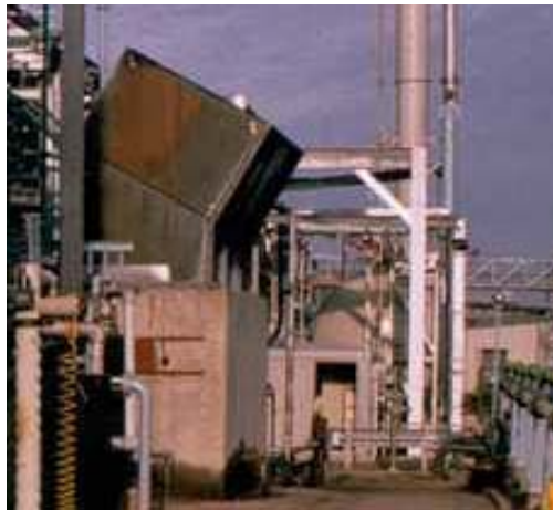
Figure 1 Ground level burning pit.
