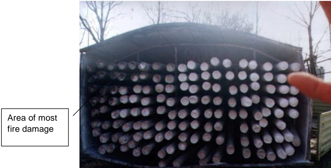
Photograph 3: Looking into underside of filter housing
