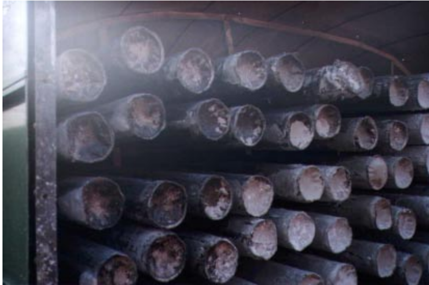
Photograph 4: Showing burning to one side of filter sock bottoms
