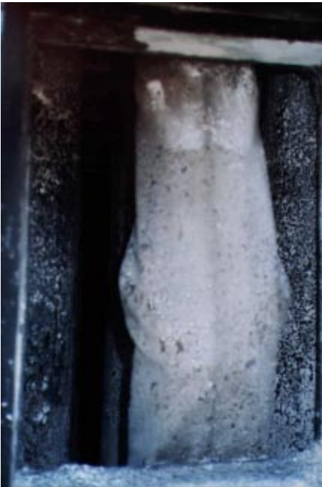
Photograph 1: Top of filter showing socks inside and damage to body and filter base (to left)
