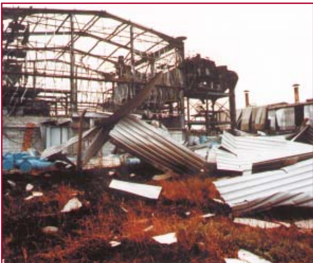
Aluminium Dust Explosion Caused by Static
