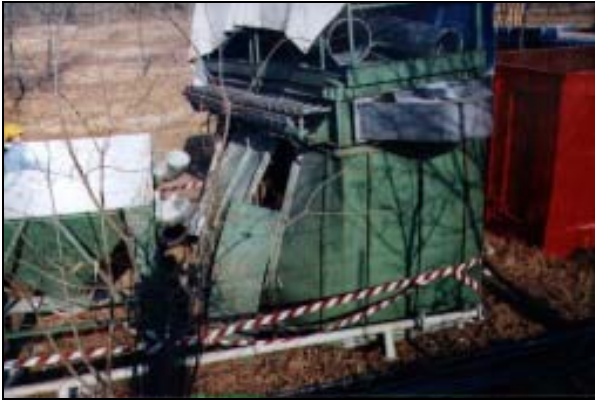
Photograph 2: Filter after explosion caused by electrostatic ignition.
